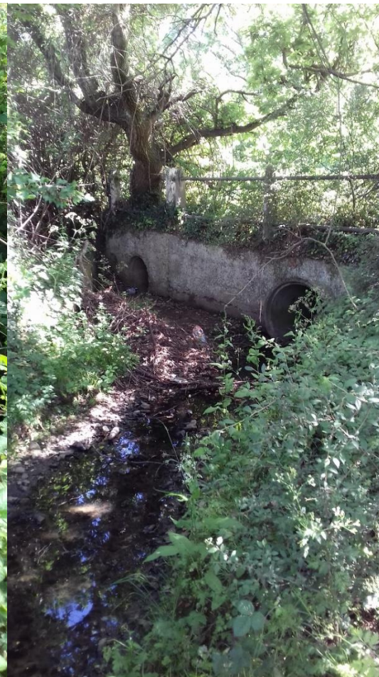
Plate 15 – Section 4, double culvert
