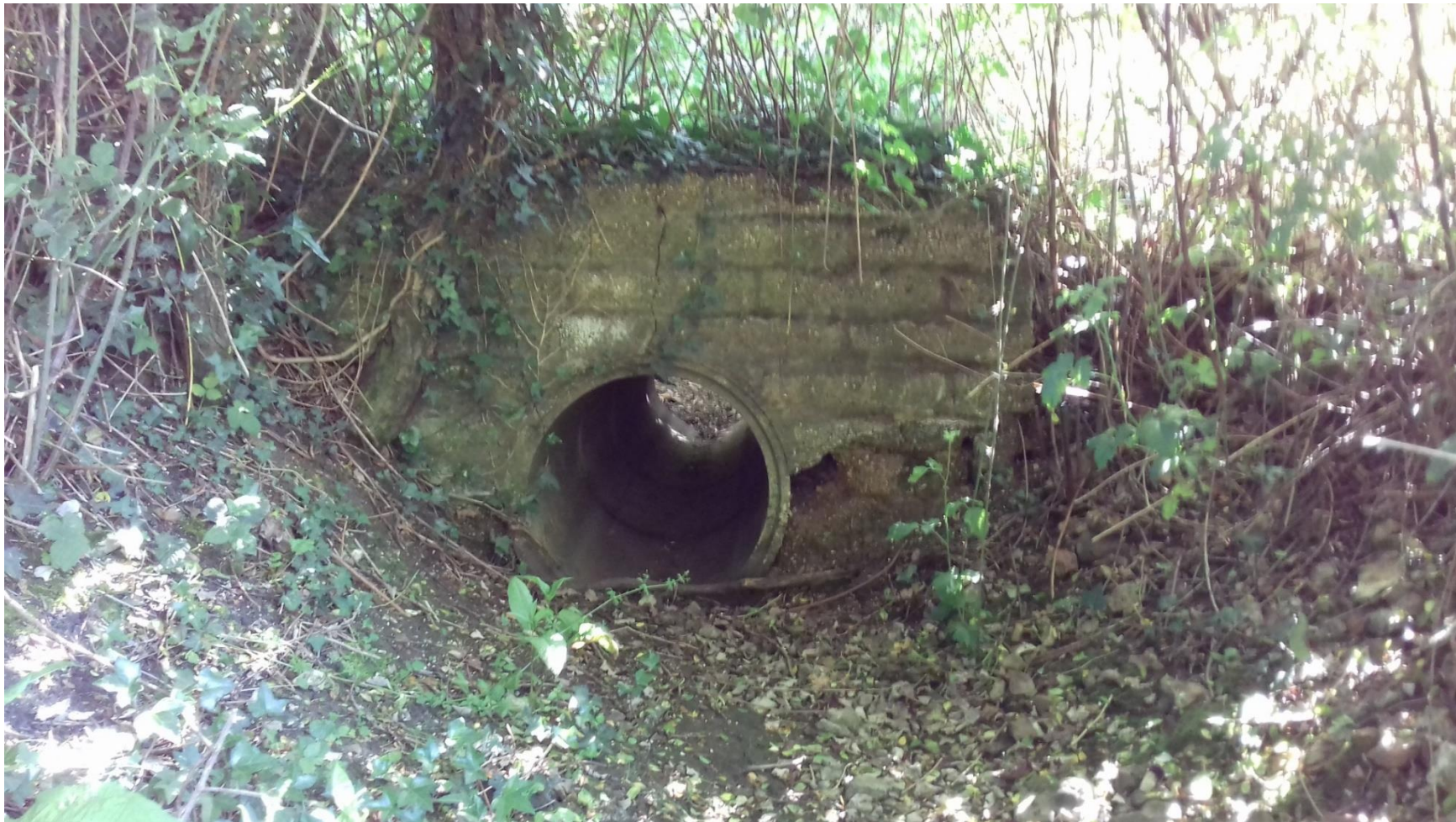
Plate 5– Section 2, northern reach. Short section of culvert.
